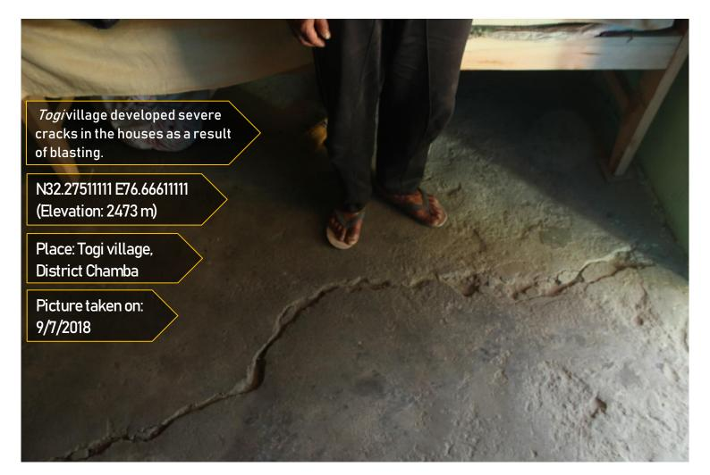
Kamla Devi's family complained of land yielding (or sinking) as a result of blasting for Bajoli-Holi HEP. In some houses the wooden logs supporting the first floor have come down because of the yielding land
